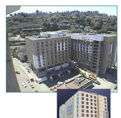
RSIC-1™ was used to control Impact Isolation Class (IIC) noise from floor to floor on 8" post tension slab concrete floors. The RSIC-1™ clips reduced the cost of this project by eliminating the need for floor finishes, allowing the owners to use stained concrete as the finish. The RSIC-1™ isolated the foot fall noise at the ceiling below the concrete slab. The RSIC-1™ clip also eliminated the high labor expense of installing a dropped ceiling below the slab.
